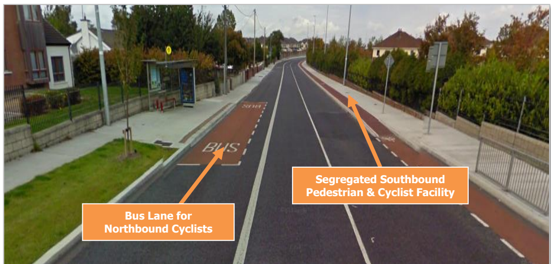
Figure 2.9: Cycling Facilities on Ballycullen Road
